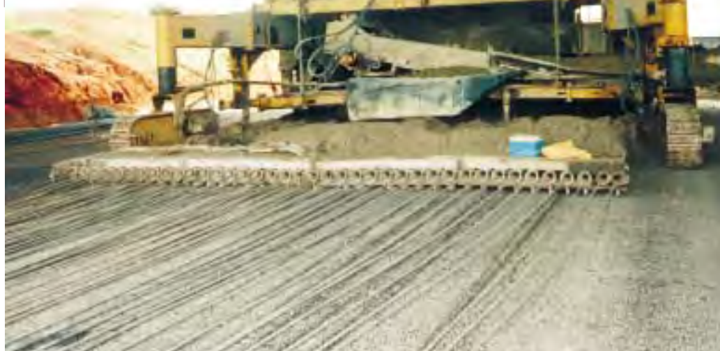
Slipform paving of the I-35 mainline.
