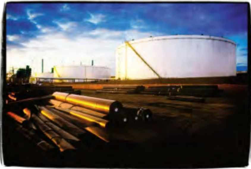
A spring sky illuminates storage tanks at the Athabasca project.
