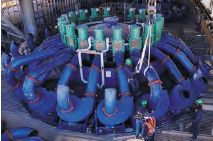
Craft workers set cyclone piping at Escondido copper project.
