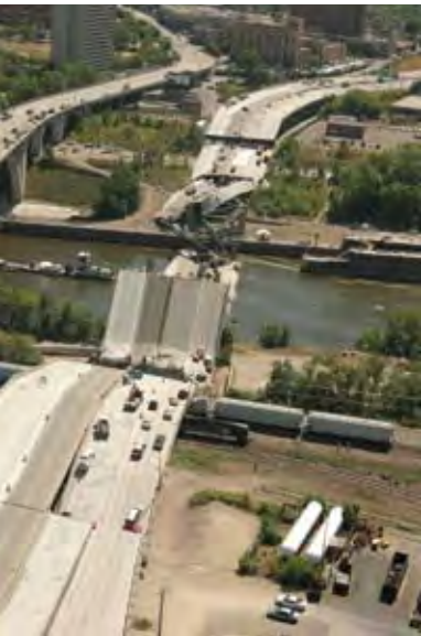
The I-35W Bridge in Minneapolis, Minnesota, collapsed into the Mississippi River and riverbanks on August 1, 2007, killing 13 people and injuring 145.
