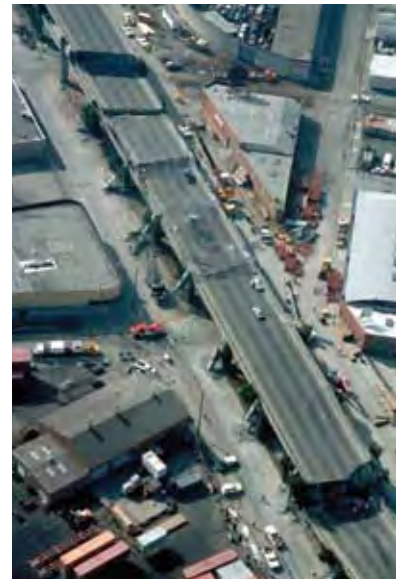
A double-deck freeway in Oakland, California, collapsed during the Loma Prieta earthquake on October 17, 1989, crushing the cars on the lower deck and killing 42 people.
