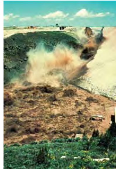
The Teton Dam in southeastern Idaho collapsed on first filling on June 5, 1976, causing the deaths of 11 people and $2 billion in damages.
